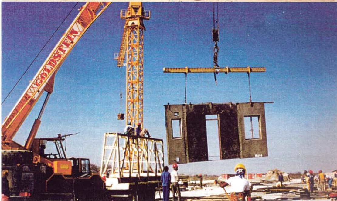
Load equalising beams, designed for the lifting of concrete panels, feature an innovative self-levelling pulley system.
